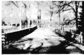
+6.27 Average response Stone wall bridge Slide #7
