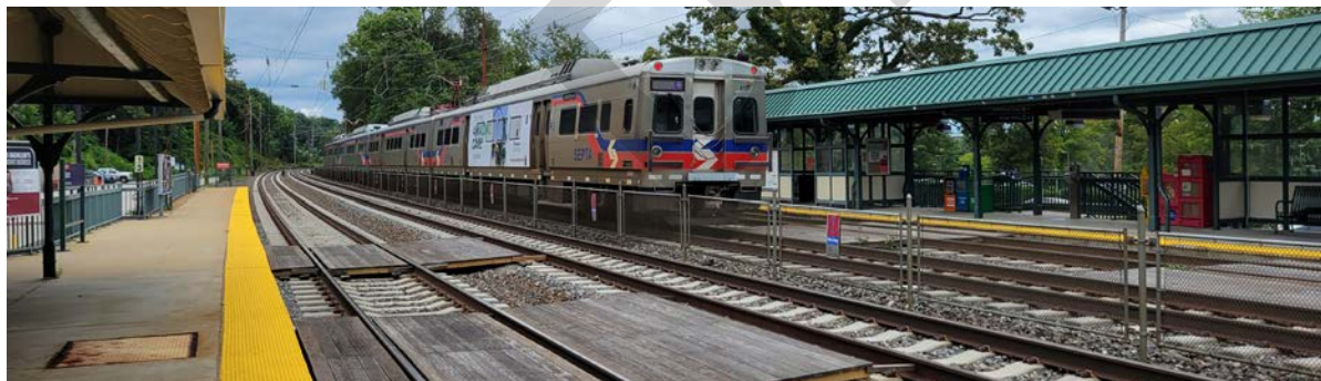
The Amtrak Keystone Corridor is a major active rail corridor in Chester County.
