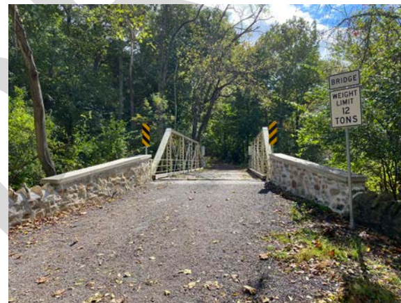
Existing bridge crossing Valley Creek.
