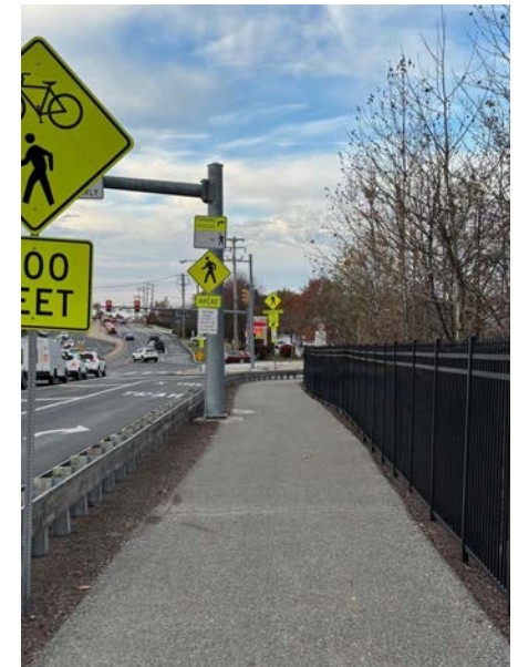
Sidepaths require a minimum 5' buffer from roads. If 5' is not feasible, vertical barriers are required to help protect trail users.
