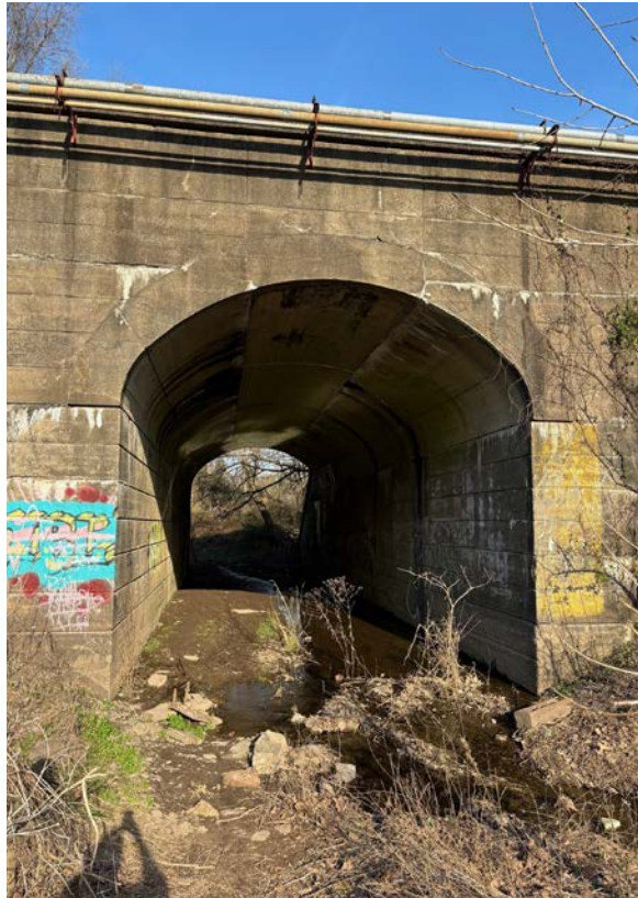
Existing condition looking east through railroad underpass.
