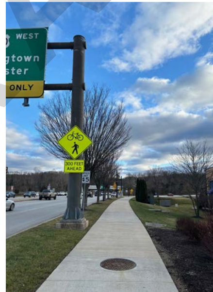
Sidepaths require a minimum 5' buffer from roads. If 5' is not feasible, vertical barriers are required to help protect trail users.
