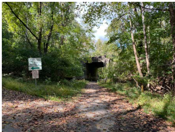
Existing tunnel beneath Pennsylvania Turnpike.
