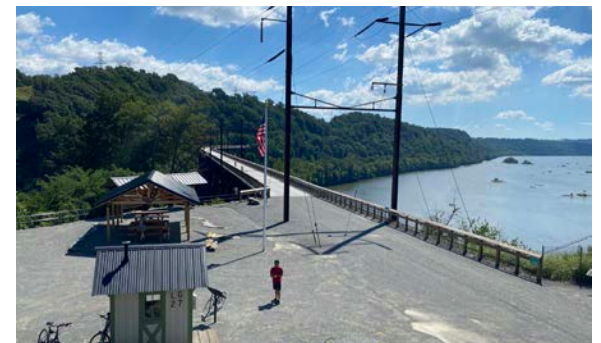
A large gathering space with various amenities was designed at the Safe Harbor Bridge along the Enola Low Grade Trail.
