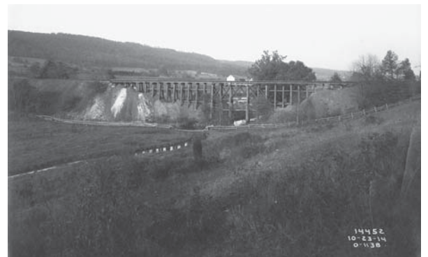
Historic photo of the Warner Spur Rail Line bridge over Valley Creek
